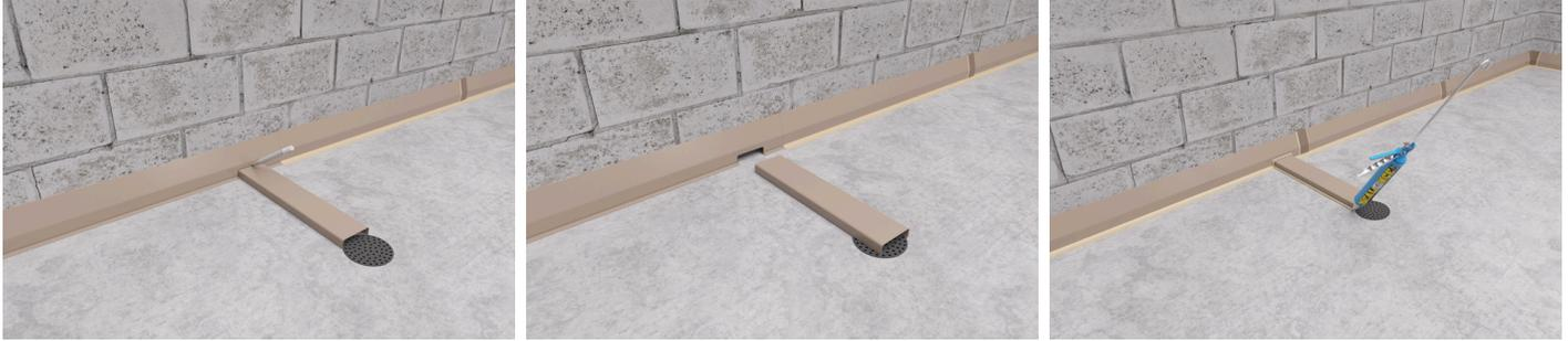
**Installing drain port:** Set the drain port in place and trace along the outside. Using a tinsnips, cut out the opening in the main section. Glue the drain port to the floor and seal the joint between drain port and main section with Pro-SealOnce Adhesive. Note: drain port does not slide into the system, it butts up to the system.
