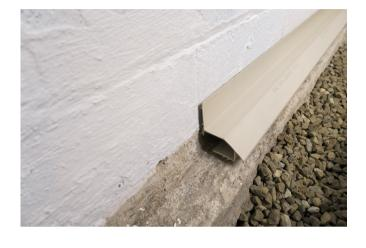
**Step 2:** Set a short section of the Drain Main on the footer to verify the back fin of the Drain Main will stick up above the floor surface 1/4" to 1" after the cement work is finished.
