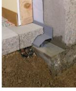
**Step 8:** Pour concrete to replace floor. Avoid pouring into inspection ports.
