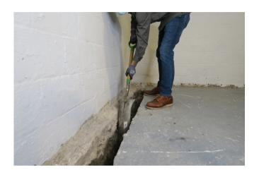
**Step 1:** The floor has to be a minimum of 3-1/2" thick over the footing. Beginning at the sump pump, remove concrete floor away from the wall approximately 6" wide and all the way down to the footer.
