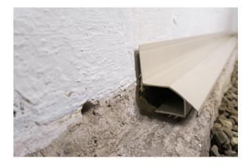
**Step 4:** Layout the Drain Main Basement System using the pre-molded corners, inspection ports and sump drop kit until you have a continuous conduit along the open trench.
