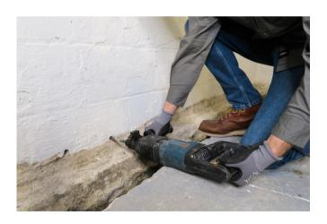
**Step 3:** Drill weep holes into empty cells in the bottom row of blocks 1/2" to 1" above footing.
