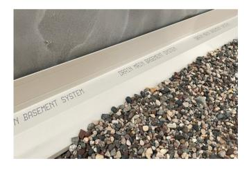
**Step 7:** Pour pea rock into the trench. Fill the trench up to the top of the footing with rock.
