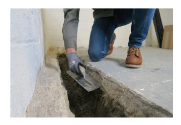
**Step 6:** Before pouring rock into trench, dig out 2" of dirt under existing concrete floor. This will help prevent moisture wicking between the concrete seams.
