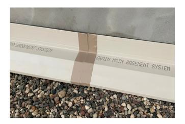
**Step 5:** Seams between the main sections should be covered with vinyl duct tape to keep concrete from getting into the system while pouring concrete.
